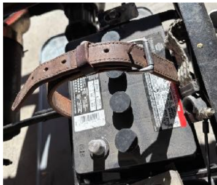
Leather belt lifter around the battery. Photo provided by Don Neidigk, February, 2025.
